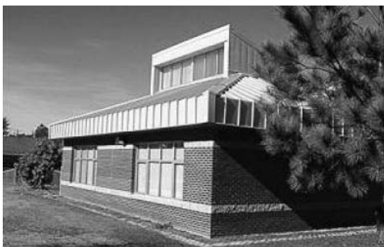
Figura 32 - Four Oaks Elementary School, EUA. Fonte: < www.innovativedesign.net >. Acesso em: 10 abr. 2006
