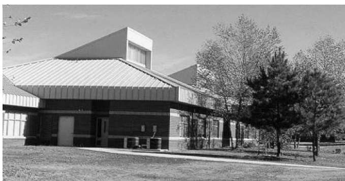
Figura 33 - Four Oaks Elementary School, EUA. Fonte: < www.innovativedesign.net >. Acesso em: 10 abr. 2006
